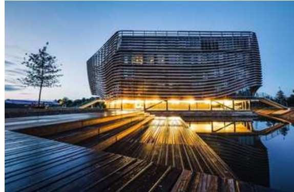
Figure 1. Wetsus building in Leeuwarden (NL).
