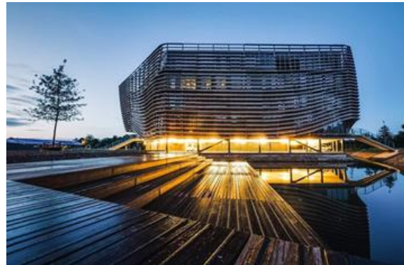
Figure 1. Wetsus building in Leeuwarden (NL).
