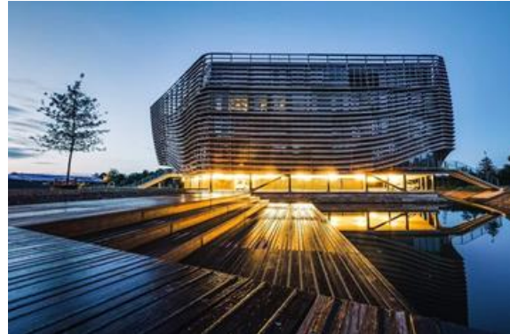
Figure 1. Wetsus building in Leeuwarden (NL).
