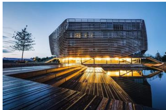
Figure 1. Wetsus building in Leeuwarden (NL).
